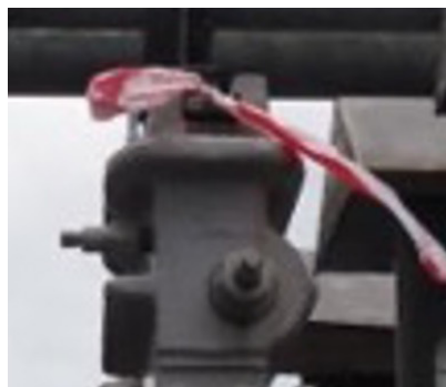
Figure 11: Example of Equipment Leak – Methane Emissions Detected From a Malfunctioning Valve on a Metering Skid
