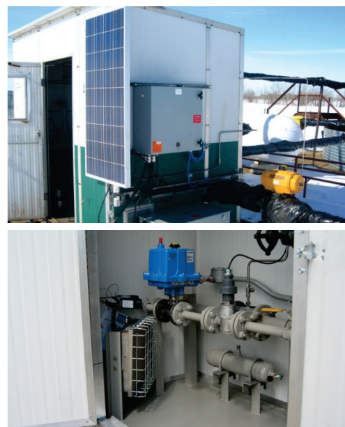
Figure 6- Calscan pictures- Bear solar control system: Top: solar panel and control panel, bottom: Electric Actuator
