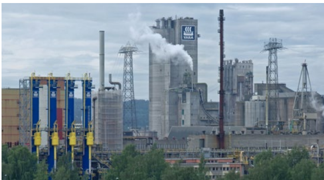
Ammonia production facility in Porsgrunn, Norway. The blue columns in the foreground remove CO 2 from the process gas; the captured CO 2 is then shipped to commercial users. Photo: Bitjungle.
