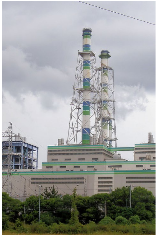
Mizushima 156 MW Coal-NH 3 boiler in Okayama, Japan (Chugoku Electric). Photo: Phronimoi.
