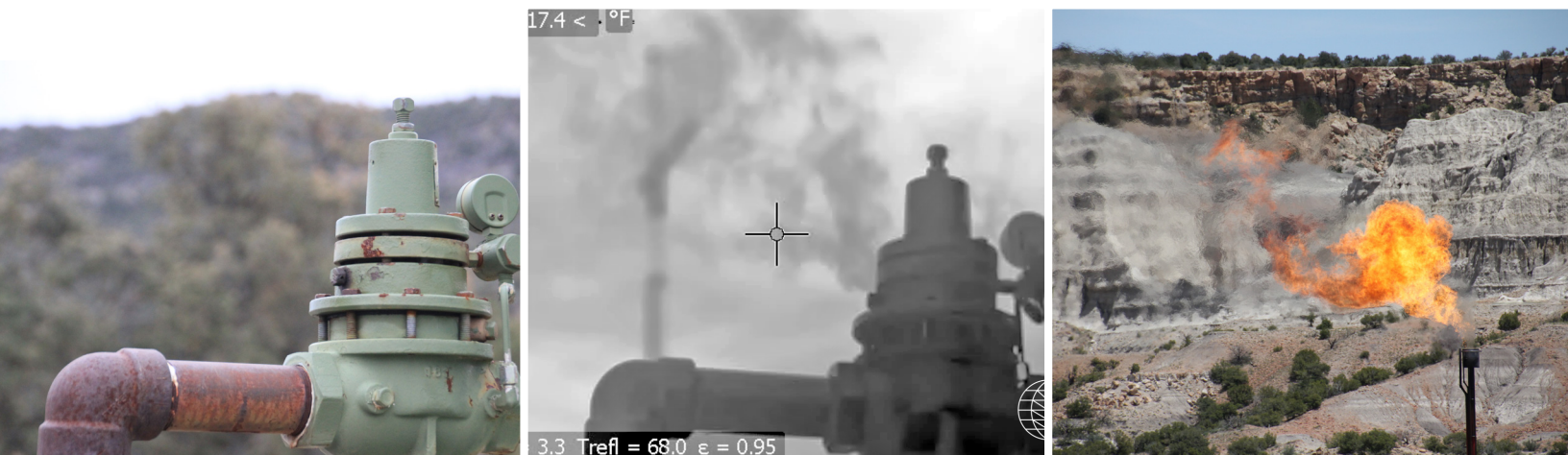
Photos: Left image shows a normal view of a San Juan County oil and gas facility. Center image is an infrared view of the same facility, showing otherwise invisible air pollution. At far right, a flare burns excess volatile organic compounds.
