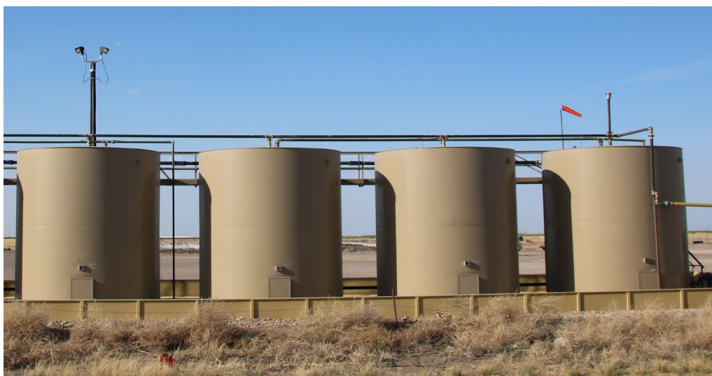
Storage tanks at a Primexx facility in west Texas in the Permian Basin. The vertical pipe on top of the rightmost tank vents methane and toxic volatile organic compounds. Go to page 15 to see an infrared view of the vented pollution.
