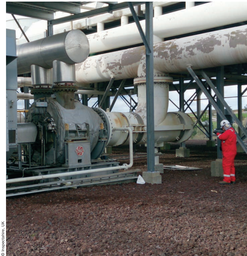
Leak detection at a natural gas processing plant. Over 400,000 metric tons of methane is leaked at natural gas processing facilities each year.
