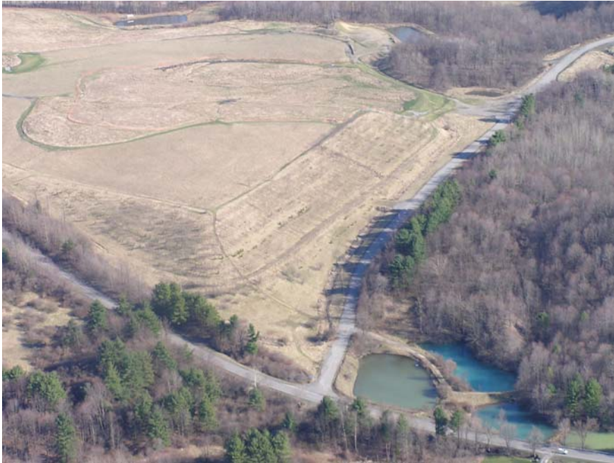
Figure 3: Aerial view of Stacks Run Refuse Site Extension
